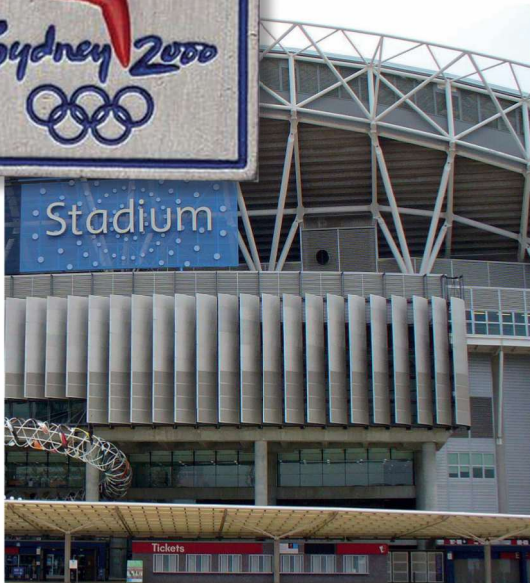
Stadium Australia Fot: Archiwum
